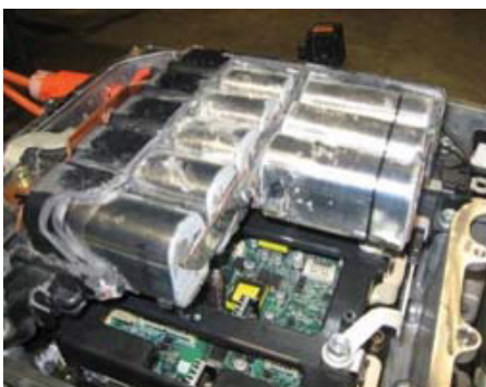
Fig. 61- Drenaje del sistema. NFPA-HEV-EV-Safety-Training-Student-Manual-1.0
