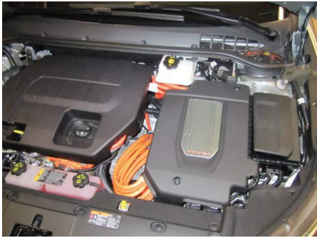
Fig. 37- Cableado interno NFPA-HEV-EV-Safety-Training-Student-Manual-1.0
